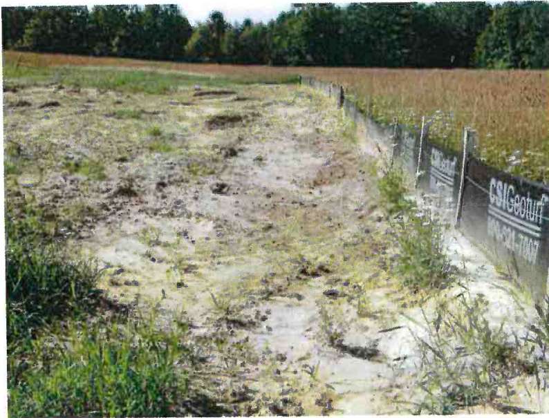
Photograph #17: Southwest corner of the GTTC property looking southerly at showing sediment/ponded area along silt fence. Taken by C. Grobbel, Grobbel Environmental & Planning, July 4, 2014.
